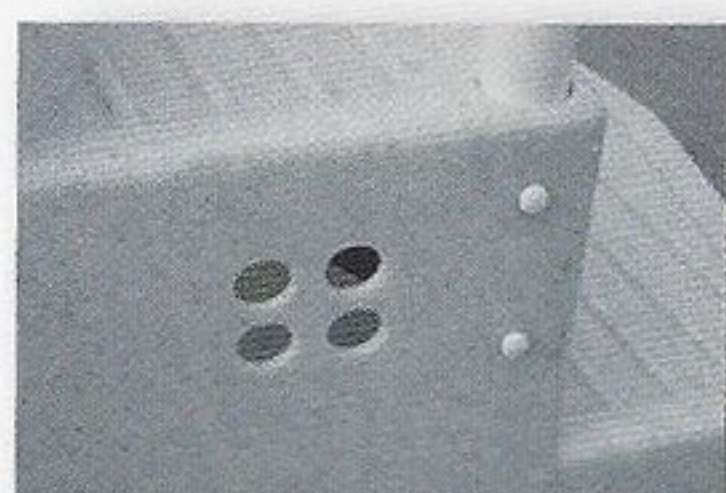
Port holes allow water to circulate through staircase.
